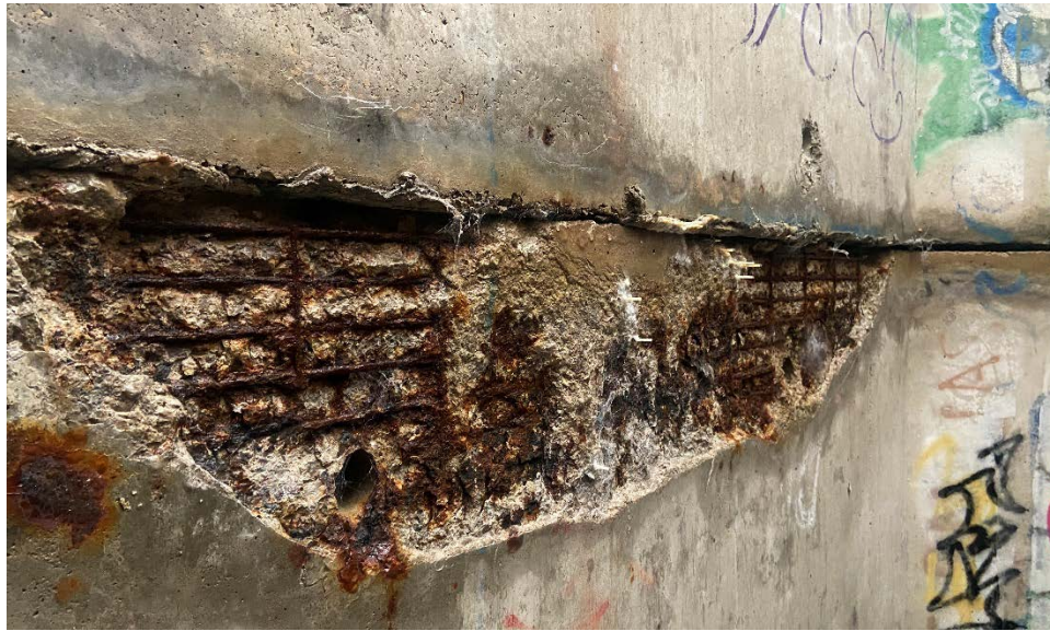
Photograph 2: Underside of the Culvert
