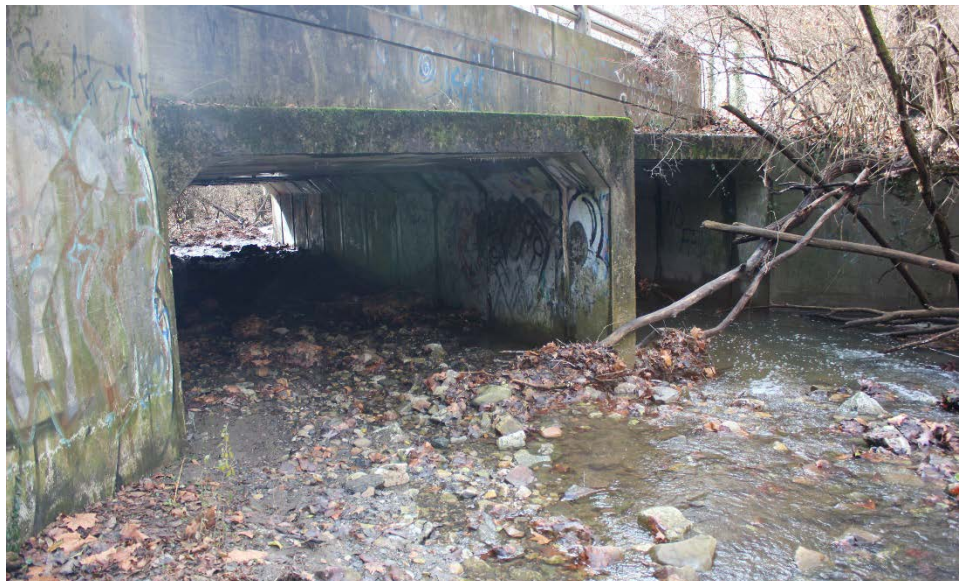
Photograph 3: Twin Box Culvert
