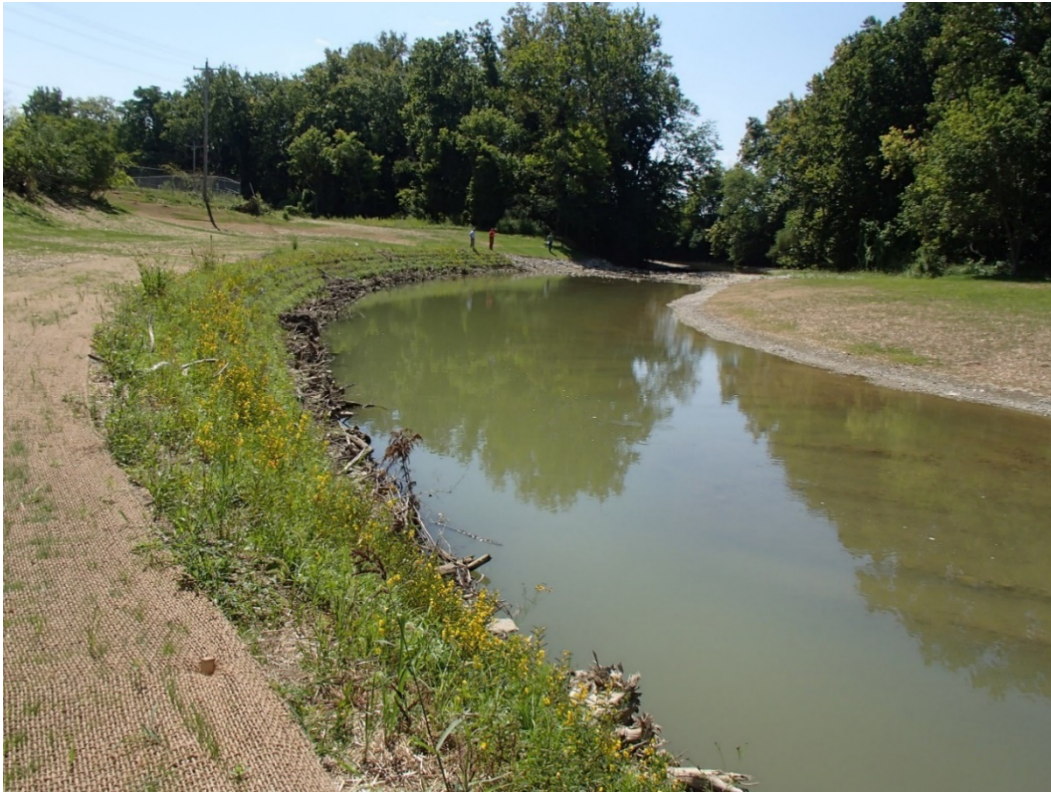
Figure 5-5: Live brush layering. Indian Creek, Butler County, Ohio
