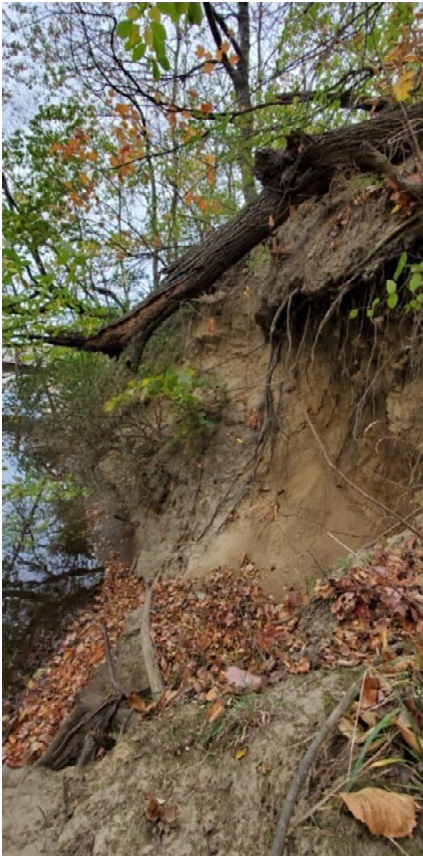
Figure 4: East Bank Severe erosion/Sloughing.
